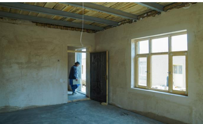
A completed shelter in Herat Zenda Jan has been handed over to an affected family after the devastating earthquake - the inside look of the construction, September 2024. (Photo: ARCS)
